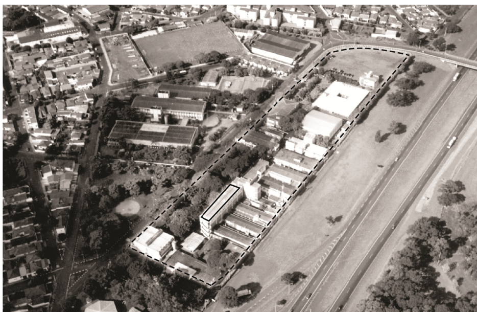
Figure 1. Aerial view of the Institute of Chemistry in 2011, the original building constructed in the 60s is highlighted in a solid line rectangle and the actual area is highlighted in a dashed rectangle (Santos & Luiz 2011)
