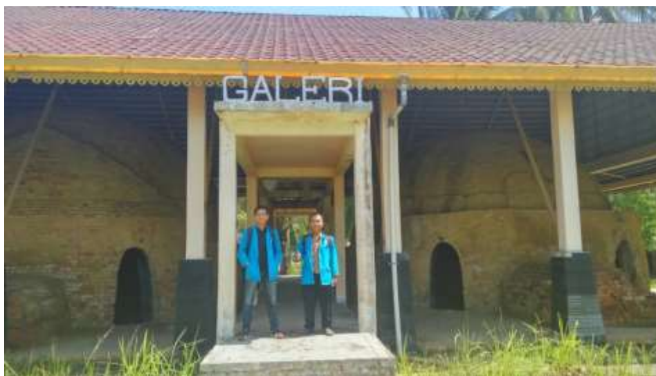
Figure 2. The Bintan Regency Government carries out conservation by building protective buildings
