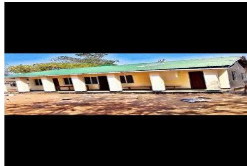
Figure 2. Appearance of Dispensary building within Kaliua District after establishment of DHFF program
